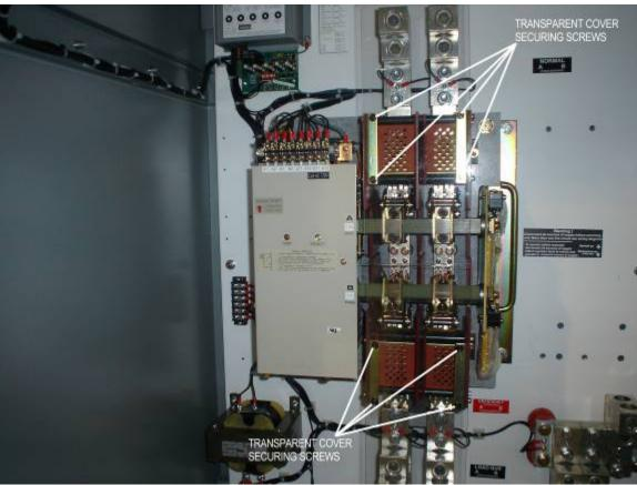
Figure 4. TRANSPARENT COVER SECURING SCREWS
